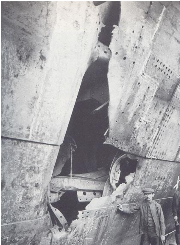
Damage to the Olympic from the HMAS Hawke impact
